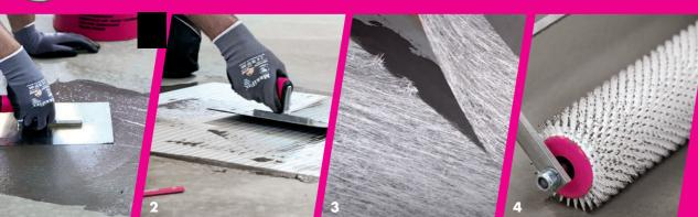
Grind the surface and remove any layers which could impair adhesion. Then apply **THOMSIT R 766** to the entire surface which has been treated.
